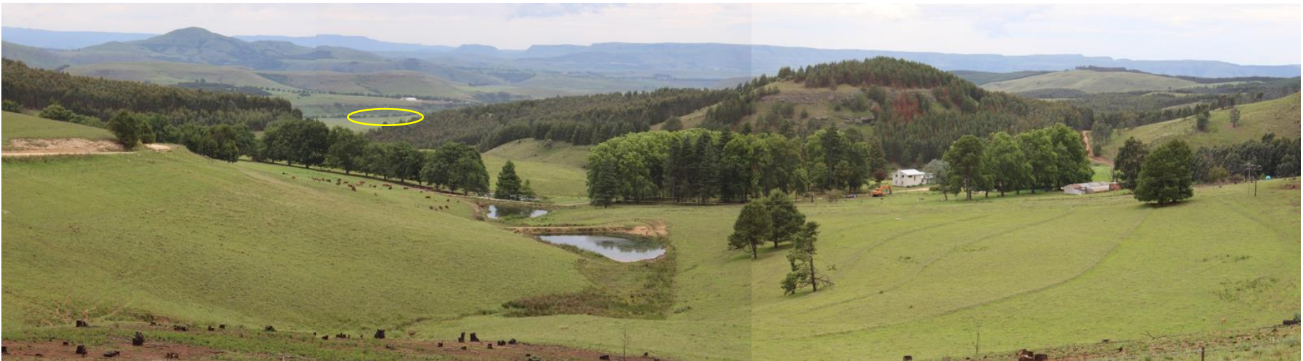
Plate 4: View towards the dam site from the P322 on the high lying southern ridge. Dam site visible and marked in yellow.
