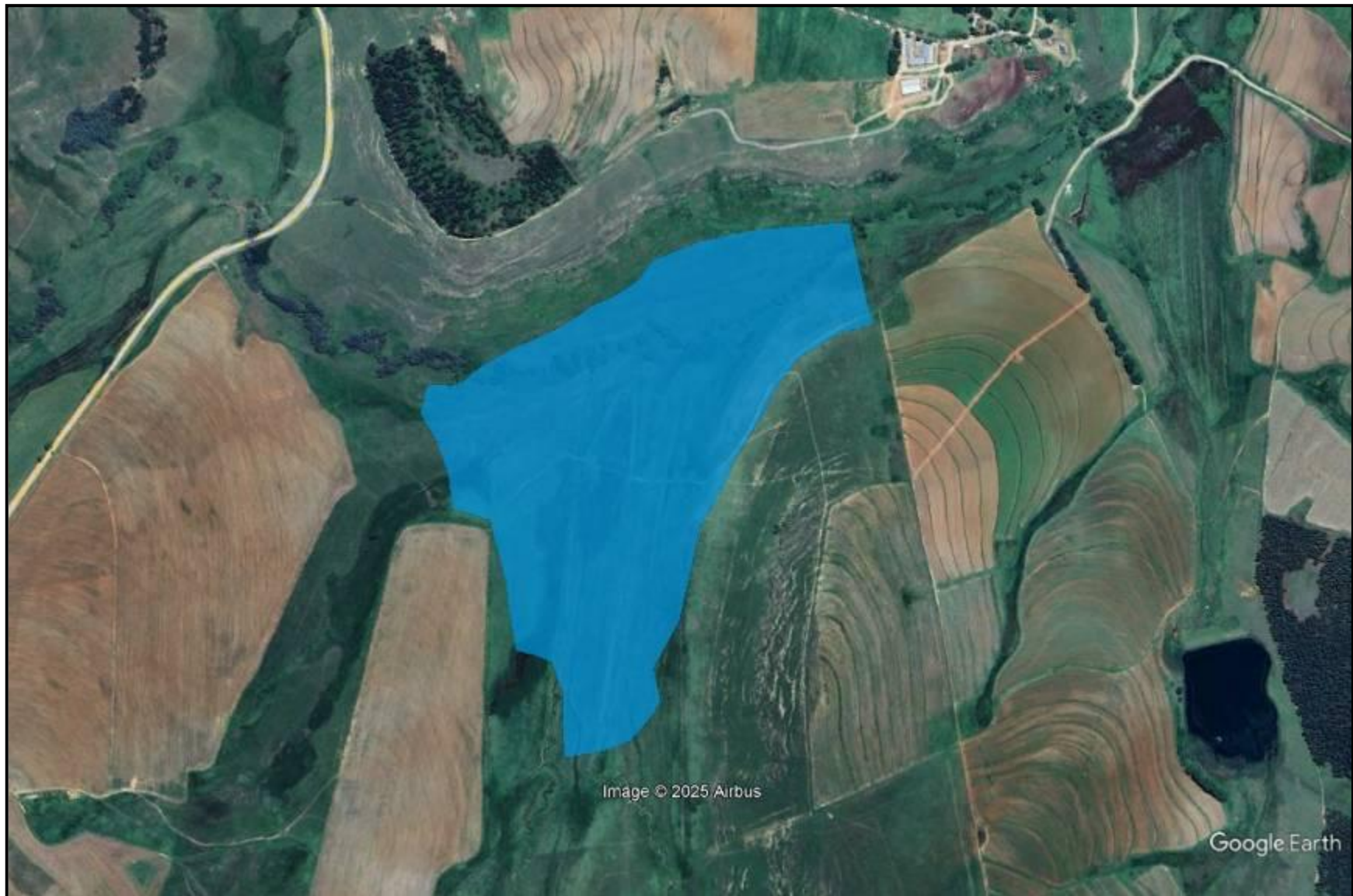
FIG. 2: AERIAL OVERVIEW OF THE DEVELOPMENT
