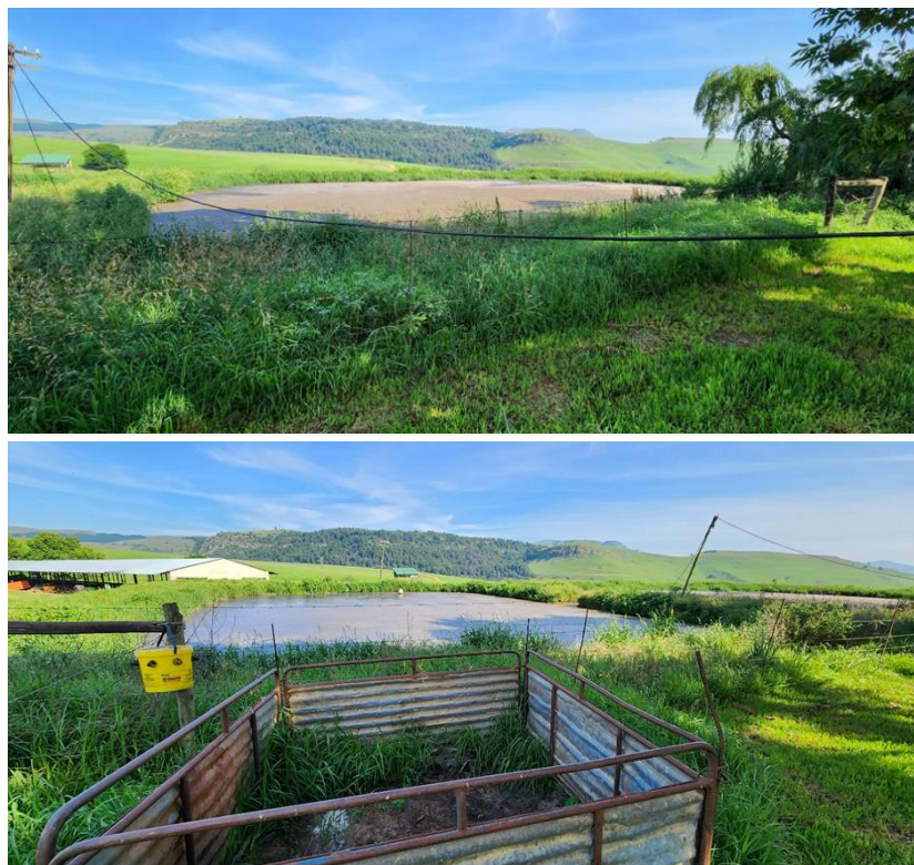
Figure 8-2: Sludge Dams with Solids and Liquids
