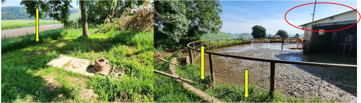
Figure 6-1: Trenches Conveying Sludge from Dairy Area to the Slurry Dams
