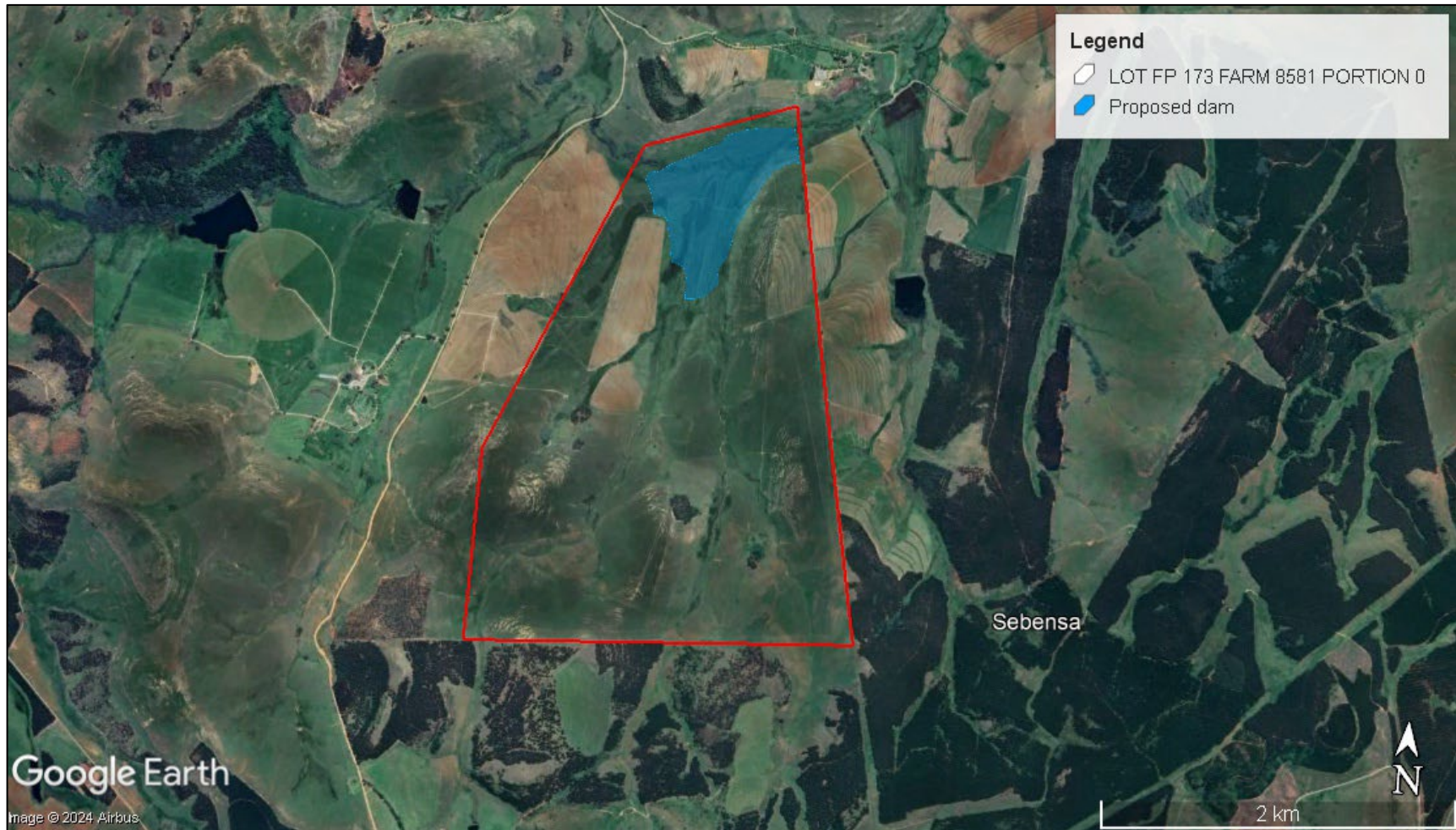
Satellite image showing the project property outlined in red, with the location of the proposed dam shaded in blue (©Google Earth Satellite Imagery).
