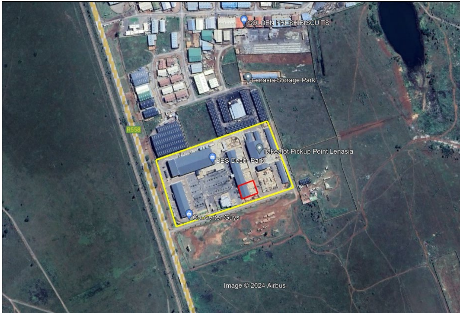
Satellite image showing the boundary of the BBS Decor Park in yellow with the location of the Platinum Blac facility in red (©Google Earth Satellite Imagery)
