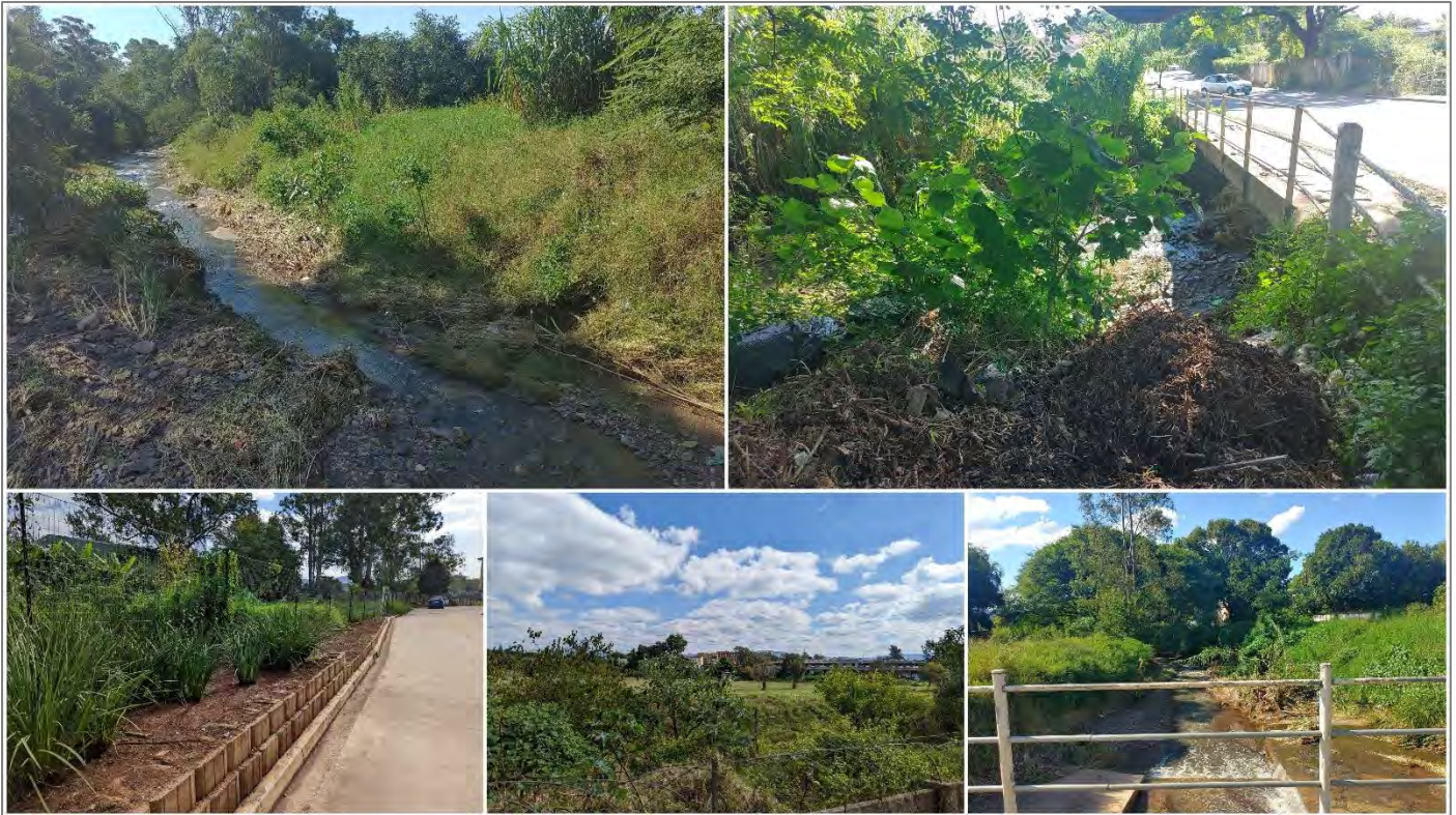
Figure 3 General site conditions and structures observed during the site visit
